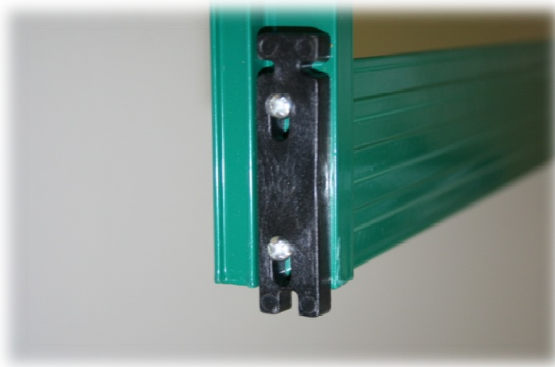
Figure 5 – Bottom of Door
