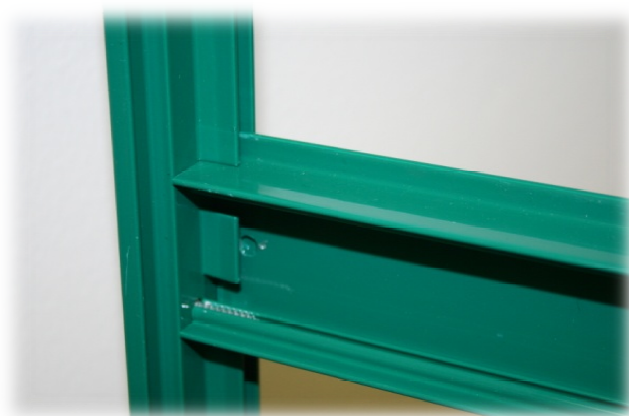
Figure 3 – Rear of Door
